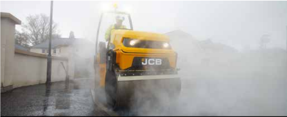
A tight turning circle makes for excellent manoeuvrability on confined sites.
